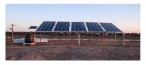
Figure 4 FCubed 5 Carocell Panel set up
