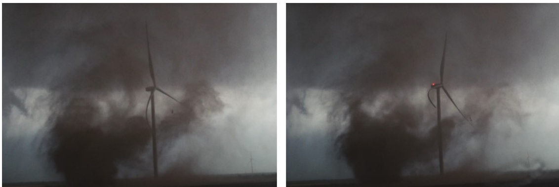
Figure 7: Wind turbine blade deflection under the influence of a storm. Figure taken from reference [1].
