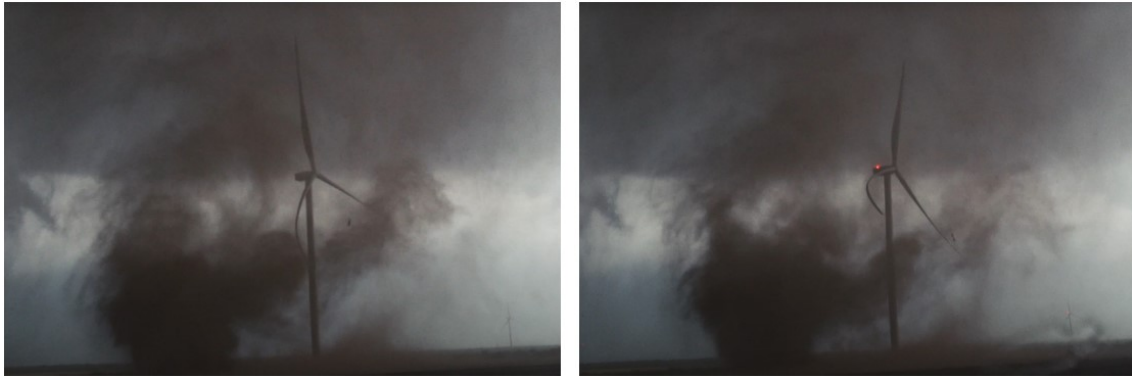
Figure 1.2: Wind turbine blade deflection under the influence of a storm. Figure taken from reference [1].
